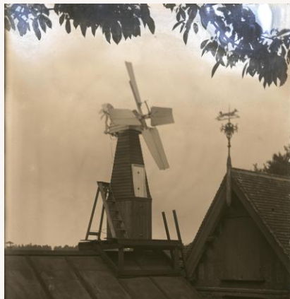
^ E Lancaster Burne's homemade mill for powering an electric light, Blackheath, 1920s (REXW-ELB-GPN-16)
