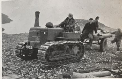
Fig. 6(b).—Hauling equipment to the site—Mynydd Anelog, North Wales.
