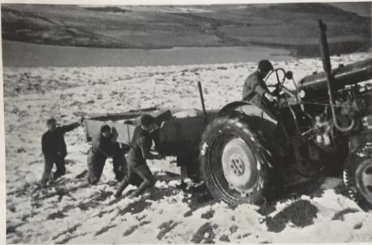
Fig. 6(a).—Hauling equipment to the site—Costa Hill, Orkney.
